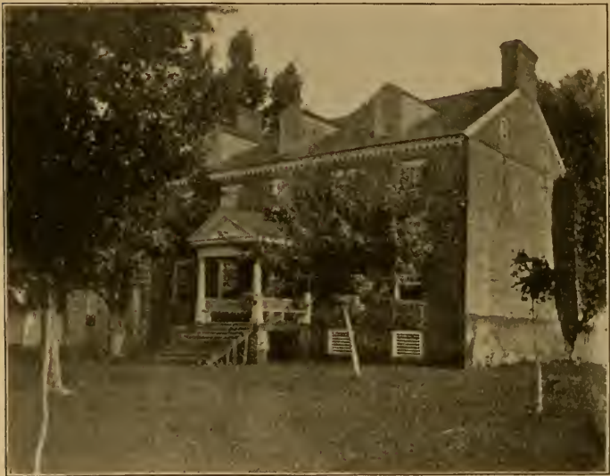
WARWICK FORT MANOR HOUSE, SECRETARY CREEK, DORCHESTER COUNTY.
